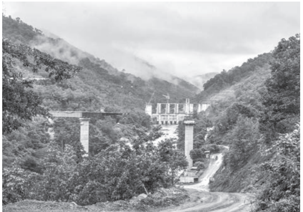
Panoramic view of Oxec hydroelectric dam. Guatemala, May 12, 2017.
